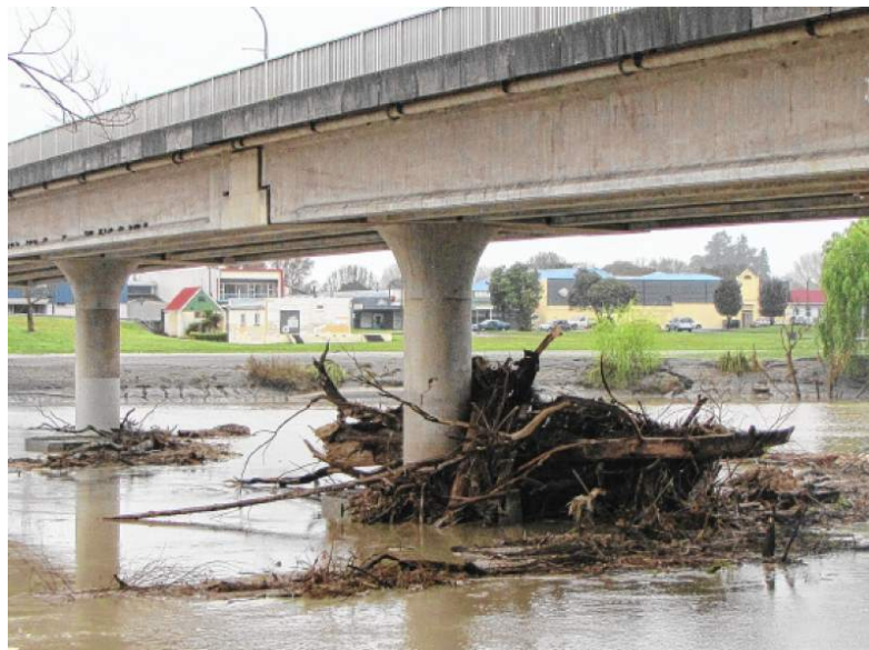
Gladstone Road Bridge blocked by forestry slash – September 2015 storm. The blockage caused flood waters to back up behind the bridge, exacerbating flooding in the Taruheru and Waimatā River upstream.
