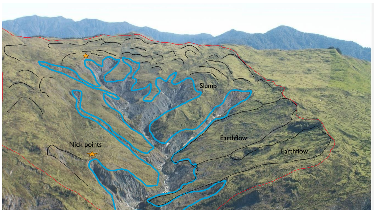
Figure 9: Multi-headed gully progressively expanding upslope towards the watershed divide.
