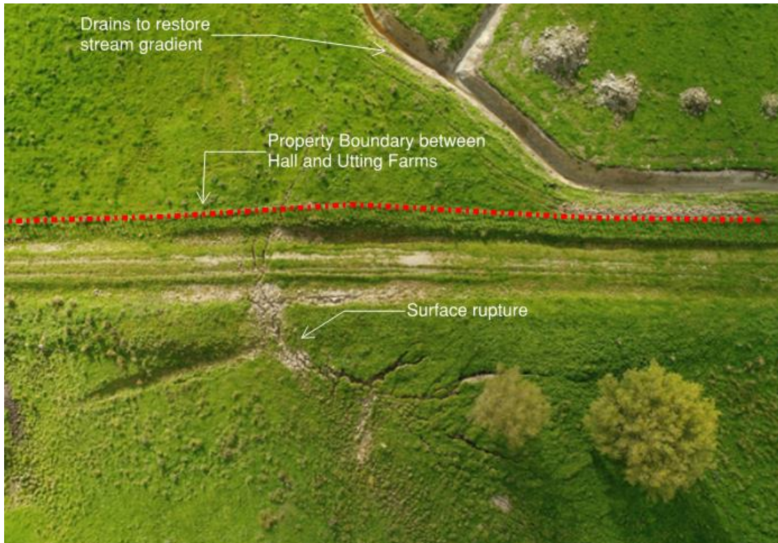
Figure 2.4: UAV image of boundary separating Utting’s and Hall’s properties showing uplift caused by Te Araroa Earthquake. Excavation works pictured were necessary to restore gradient of blocked stream.
