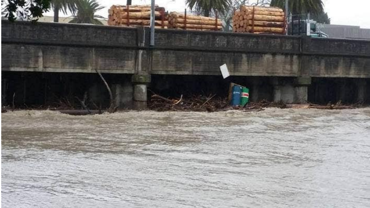
Figure 2.5 Debris gathering of the Taruheru River under the Gladstone Road bridge, Gisborne. (Gisborne Council, 2015).
