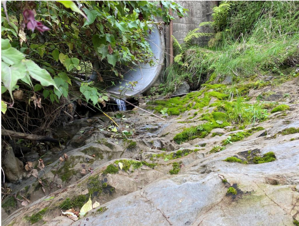
Figure 17. A perched culvert present in the Makahakaha Stream tributary in Waimanu Forest, 3 April 2023
